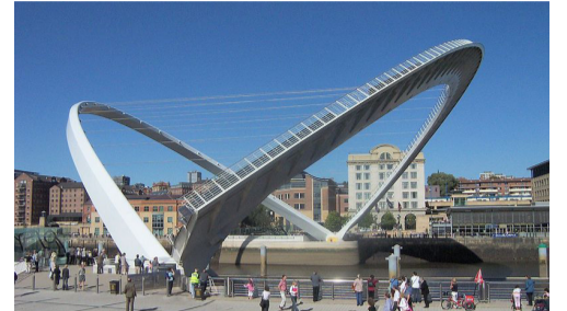
Millennium Bridge in Gateshead, England
